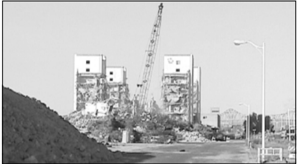
Demolition at Building 313 to make way for Port of Oakland redevelopment.
