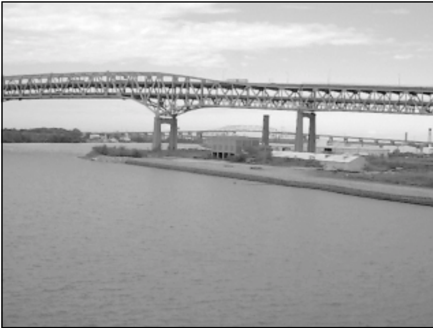
The Girard Point Management Area, historically used as an active incinerator and landfill, showing a portion of river bank that has undergone stabilization.
