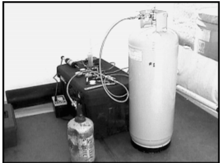
Contents from a damaged unearthed ethylene oxide cylinder at NSA Mid-South are transferred in a negative pressure tent prior to shipment.
