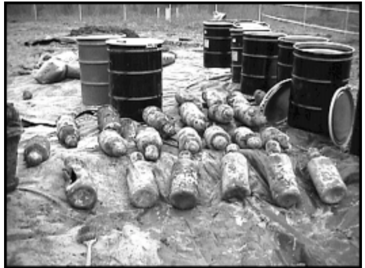
Unearthed ethylene oxide cylinders at NSA Mid-South are staged prior to transfer and disposal operations.
