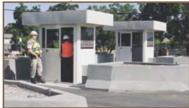
Additional security measures on East Avenue.
