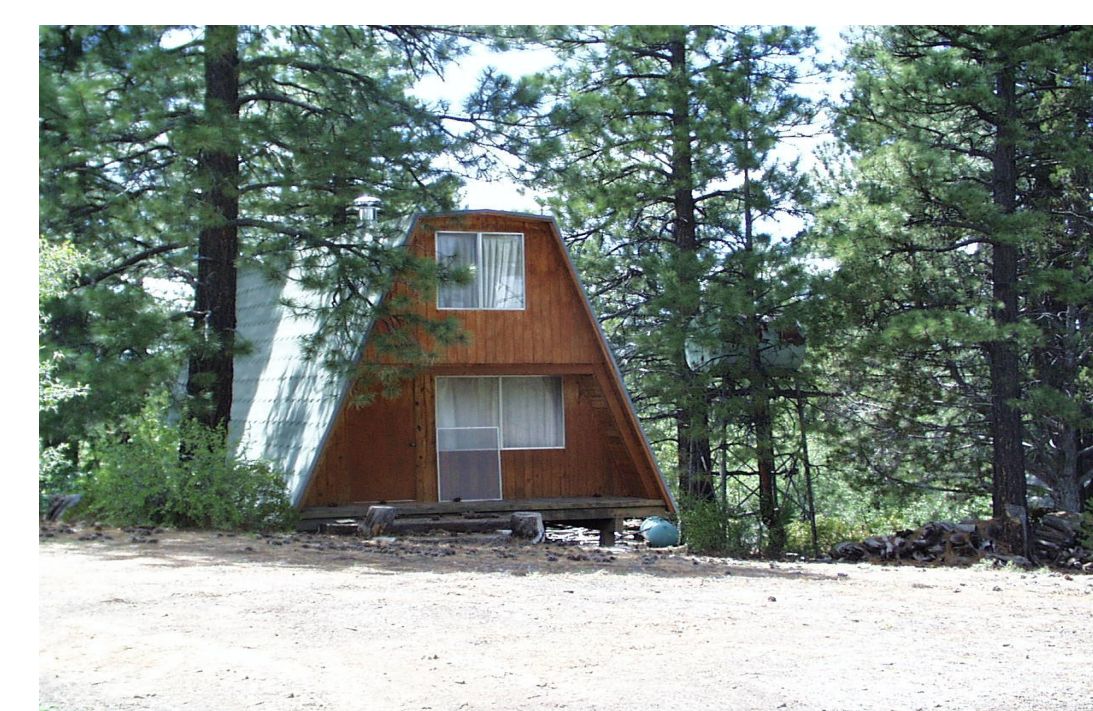
Structure near park boundary
