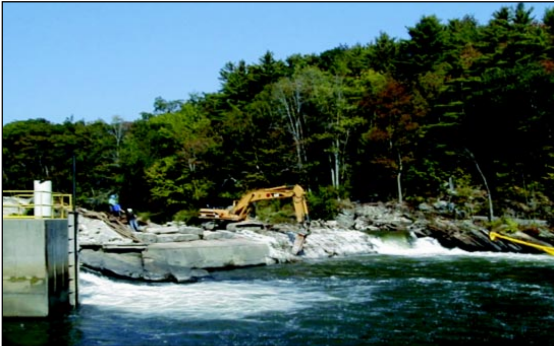
Removal of Smelt Hill Dam began in September 2002.
