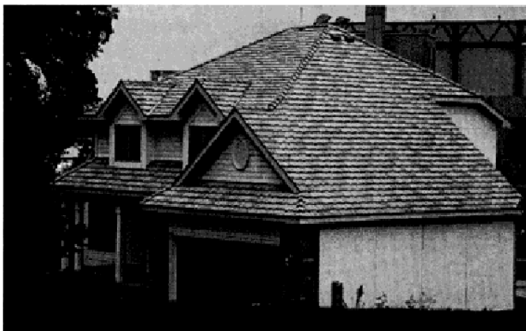
Figure 5. Experimental house at FPL roofed with wood–thermoplastic roofing shingles and currently under long-term field monitoring for durability, color stability, and UV weathering.
