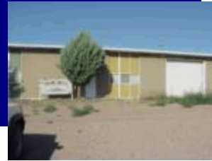
H Marker Facility
