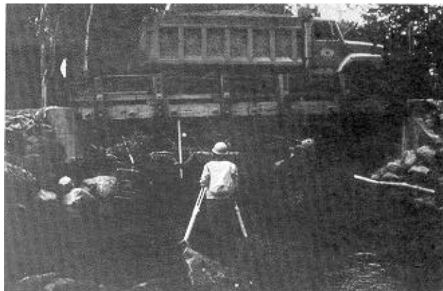
Figure 15—Measuring bridge deflection with surveyor's rod. (M92 0009-9)
