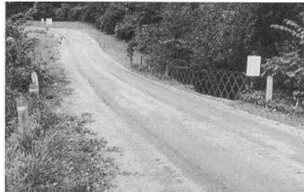
Figure 2—Original Cooper Creek bridge constructed in the 1940s.
