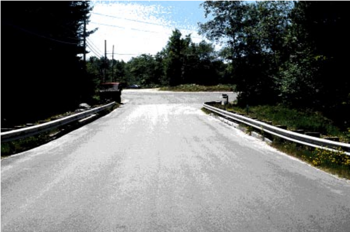
Figure 6—Completed Sanborn Brook bridge.
