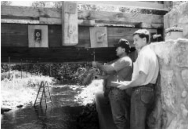
Figure 7—Measuring moisture content with an electrical-resistance moisture meter.
