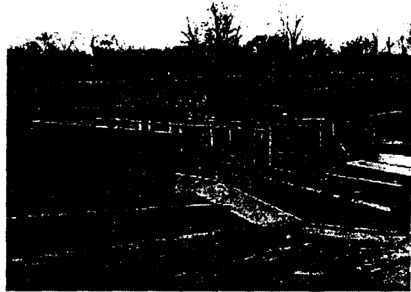
Figure 1—Construction of a stress-laminated deck by placing single laminations with butt joints on scaffolding supports.
