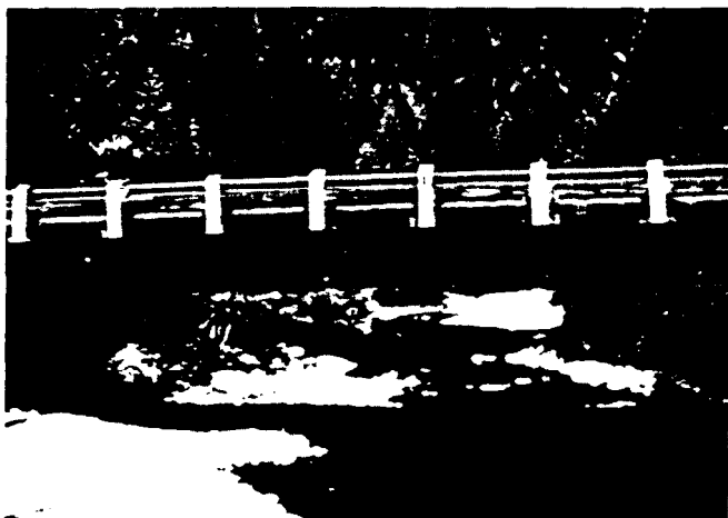
FIGURE 1 Glued-laminated timber bridge.
