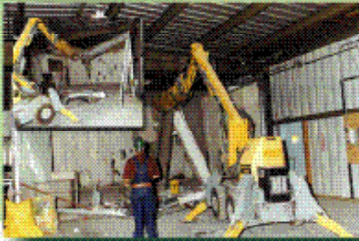
Demolition activities at WERF incinerator
