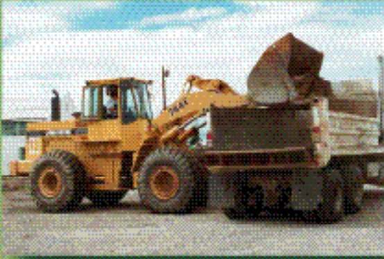
Remediation at the CFA Transformer Yard
