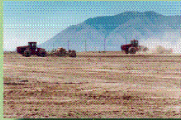
Construction activities at INEEL CERCLA Disposal Facility
