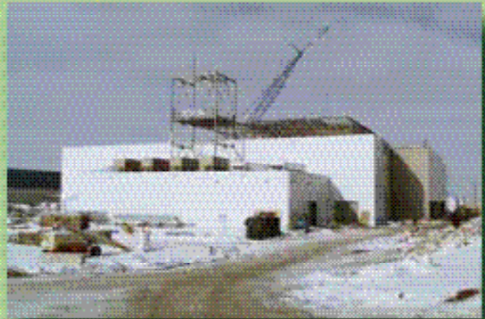
Advanced Mixed Waste Treatment Project construction is nearly complete
