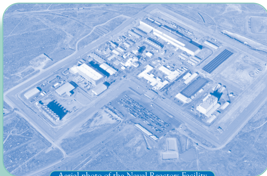
Aerial photo of the Naval Reactors Facility
