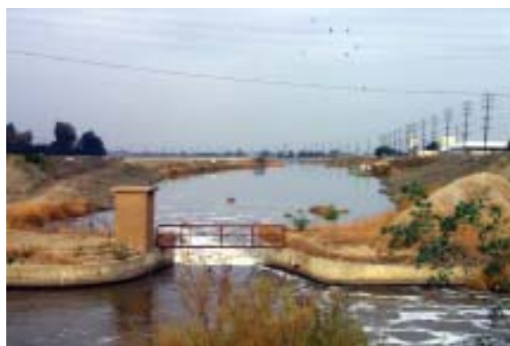
Recharge facility in the Coastal Santa Ana Basin (photograph by Carmen Burton, U.S. Geological Survey).
