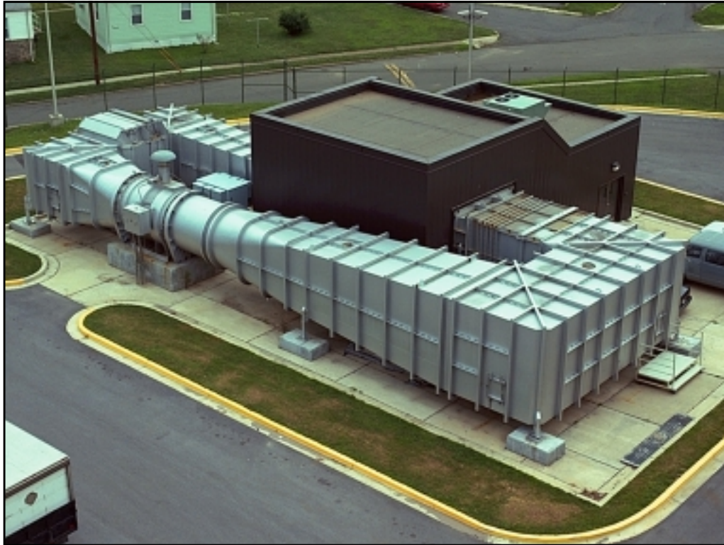
Off-Board Test Platform
