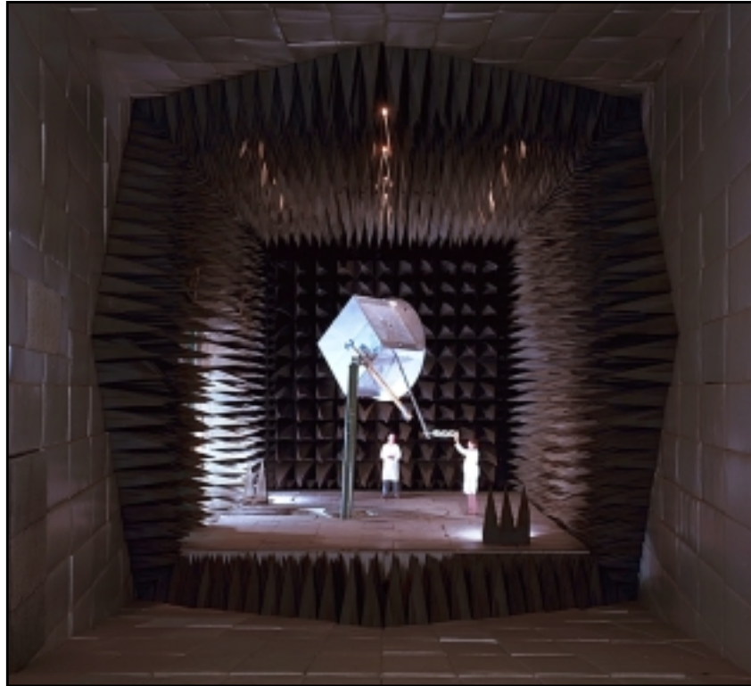
Radio Frequency Anechoic Chamber Facility
