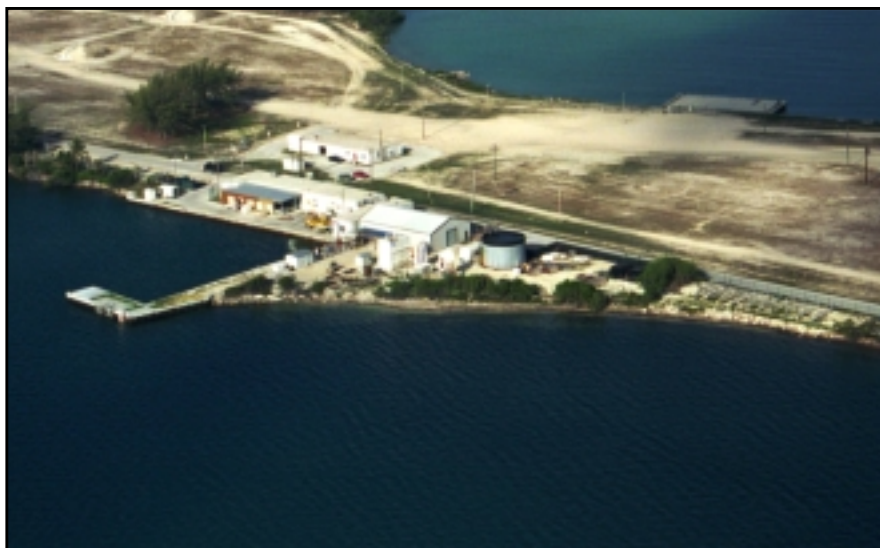
Marine Corrosion Facility
