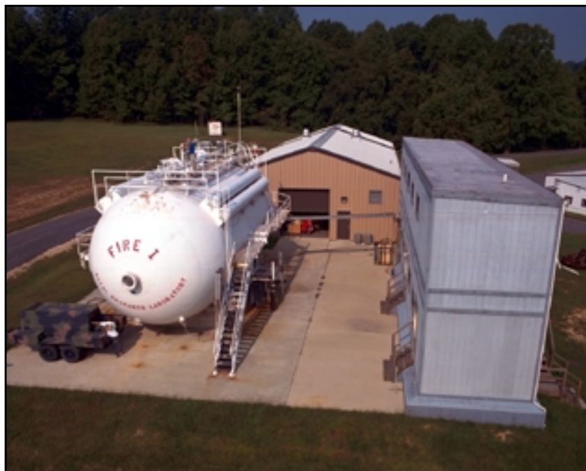
Submarine Fire Research Facility (FIRE I)
