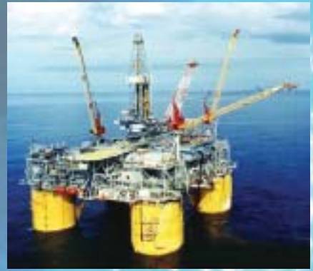
The Tension Leg Platform, Ursa, in the Gulf of Mexico
