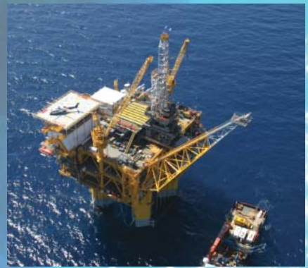
Spar production platform in the Marco Polo field located 150 miles off the Louisiana Coast in 4,300 feet of water depth.
