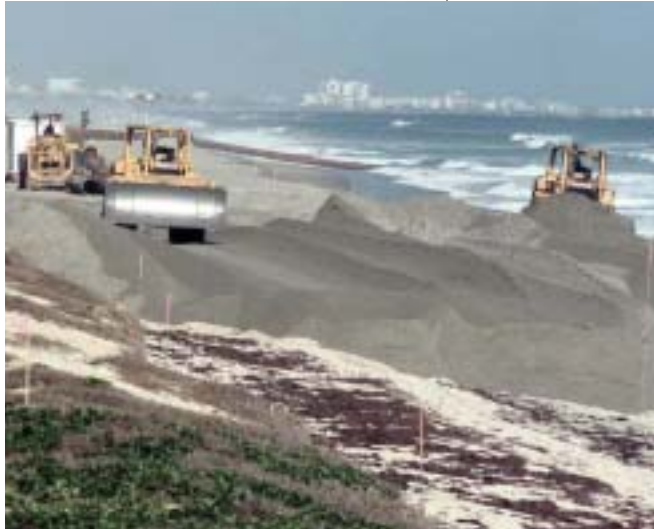
Above left: Distributing dredged sand along the beach at Patrick Air Force Base, Florida. Above right: Aerial view of beach nourishment at Patrick Air Force Base, Florida. Bottom: Sand entering a hopper dredge.
