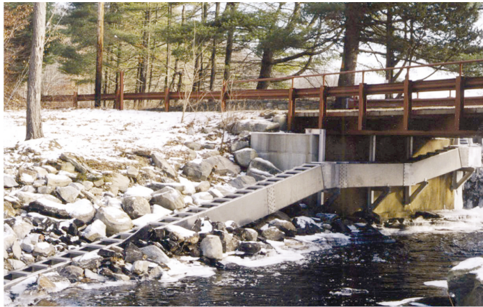
The Ed Bill's Pond project in Connecticut constructed a fish ladder to enhance migratory fish habitat.
