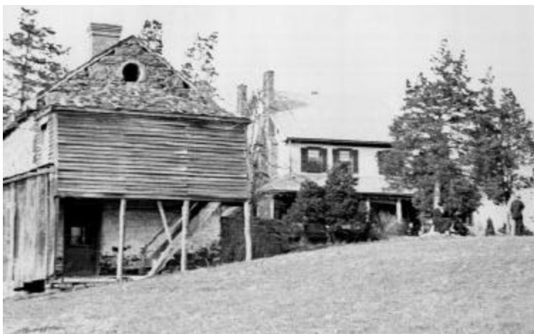
Sully south yard showing stone dairy to the left in the foreground and the main house in the background. Courtesy Elizabeth A. Crowell.
