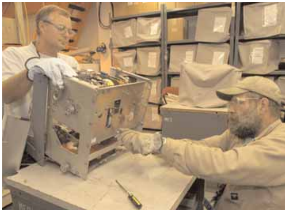
Multi-skill B Electricians Jerry Newman (left) and John Anderson refurbish a circuit breaker used on the turbine building common board at Sequoyah Nuclear Plant.
