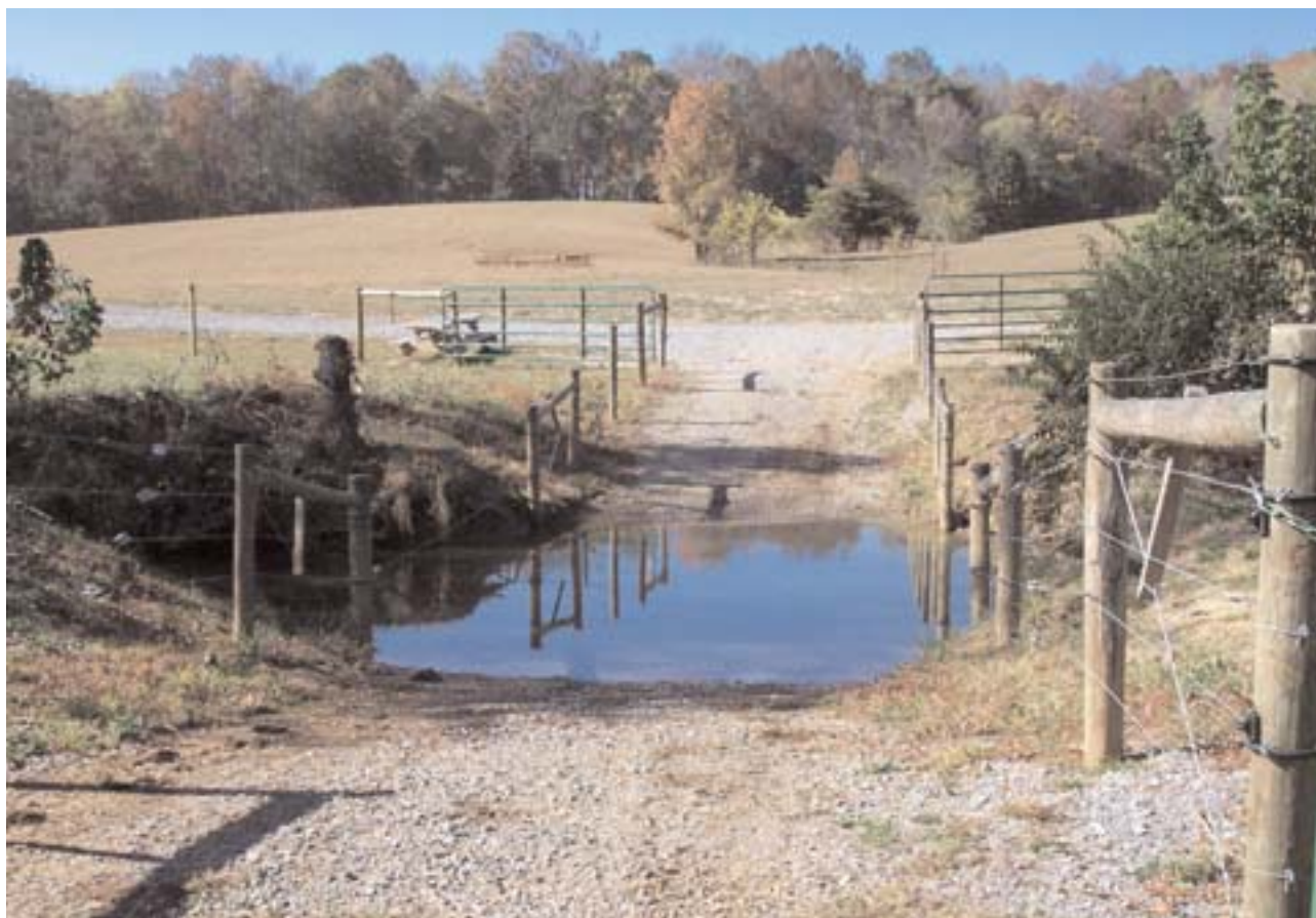
A stream crossing on Ellejoy Creek is a conservation practice that provides stable and protected areas where livestock can drink and cross streams. Fences exclude animals from all areas except the crossing. Paths are constructed using geotextile fabric and gravel to protect them from erosion.
