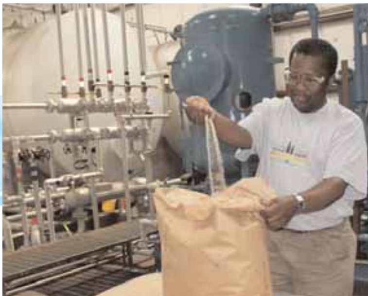
ABOVE: Electrician Foreman Mac Butler runs a sand-like substance called "Fullers Earth" through his fingers. The sand is placed in a tank to filter used oil from the generating and transmission units. "We bring in the oil in tanker trucks, pump it through the sand and put the refurbished oil into storage tanks for later use at the plants," Butler says. "We have eight storage tanks that hold 10,000 gallons each."
