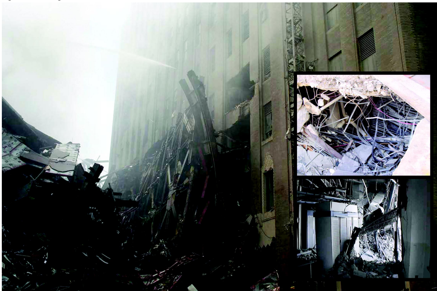
Figure 7: Damage to Verizon Central Office at 140 West Street
