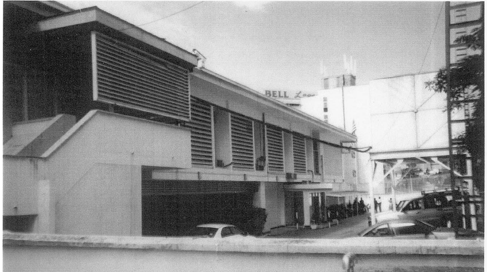
Figure 2: Existing Embassy in Kampala, Uganda
