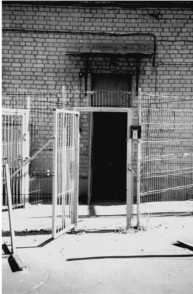
Figure 3: Gate Left Open and Unattended at a Russian Nuclear Facility
