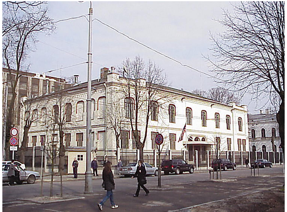
Figure 6: Insufficient Setback at a U.S. Embassy
