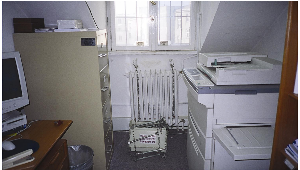
Figure 11: Chain-link Ladder Serves as Fire Escape for 6 th Floor Embassy Employees
