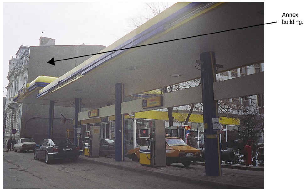
Figure 7: Public Gas Station Behind an Embassy Building Poses Security Concern
