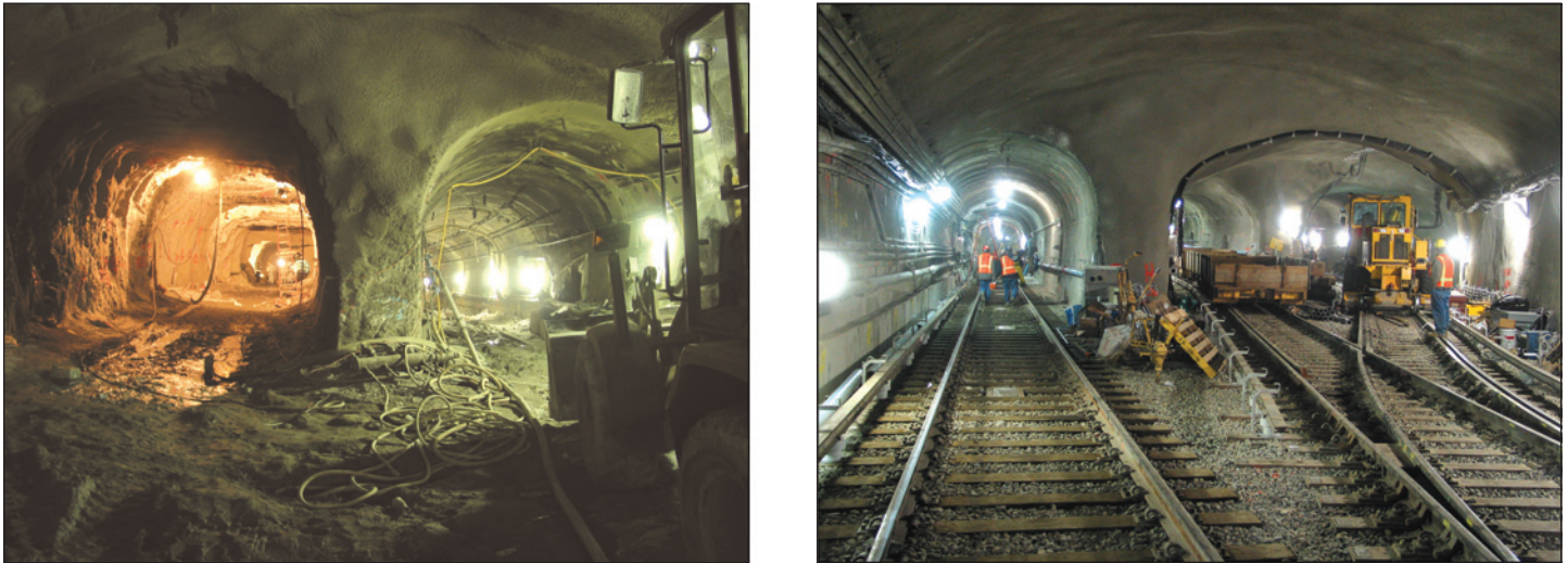
Figure 10: FEMA Funded Efforts to Remove Debris from the PATH Tunnel
