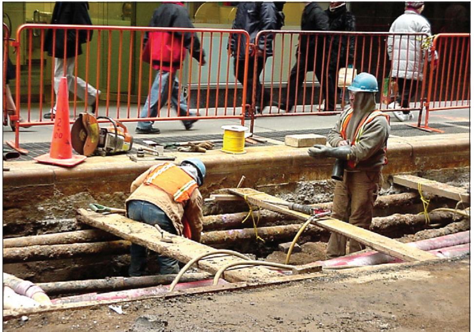
Figure 19: Workers Conducting Street Repairs in Lower Manhattan
