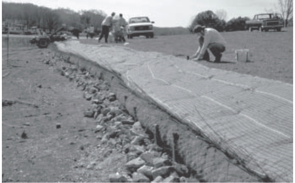
Vegetated Geogrid and Coconut Fiber Roll
