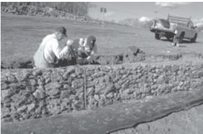
Gabions and Filter Fabric
