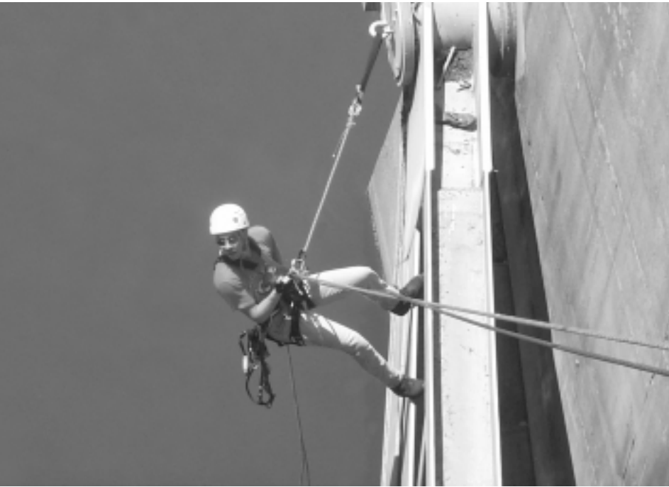
An engineer on TVA's Rope Access Team rappels down a spillway bay at Nickajack Dam in order to check the condition of the gate. Inspection crews operate in three-person teams, each member of which has completed a minimum of 40 hours of training and passed a test administered by outside instructors. Team members must undergo a two-day recertification process every year to keep their skills current.
