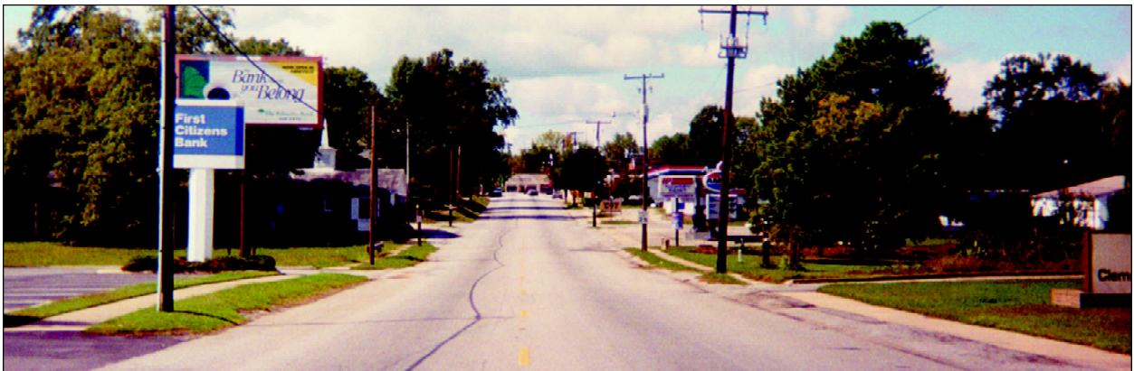
Existing 2-lane Savannah Street through Calhoun Falls.
