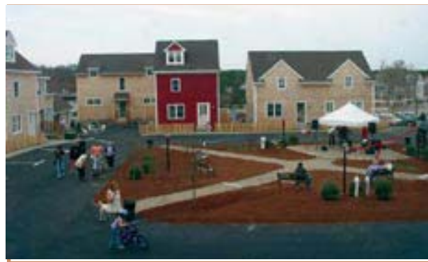
Provincetown Community Housing is an 18-unit rental project in Provincetown, MA, developed with an equity investment from the Massachusetts Housing Equity Fund.
