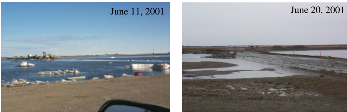
Figure 3-5. Kuparuk River causeway/bridge (eastern segment of river) shown under water during peak flow on June 11, 2001 and then high and dry and rebuilt on June 20, 2001.
