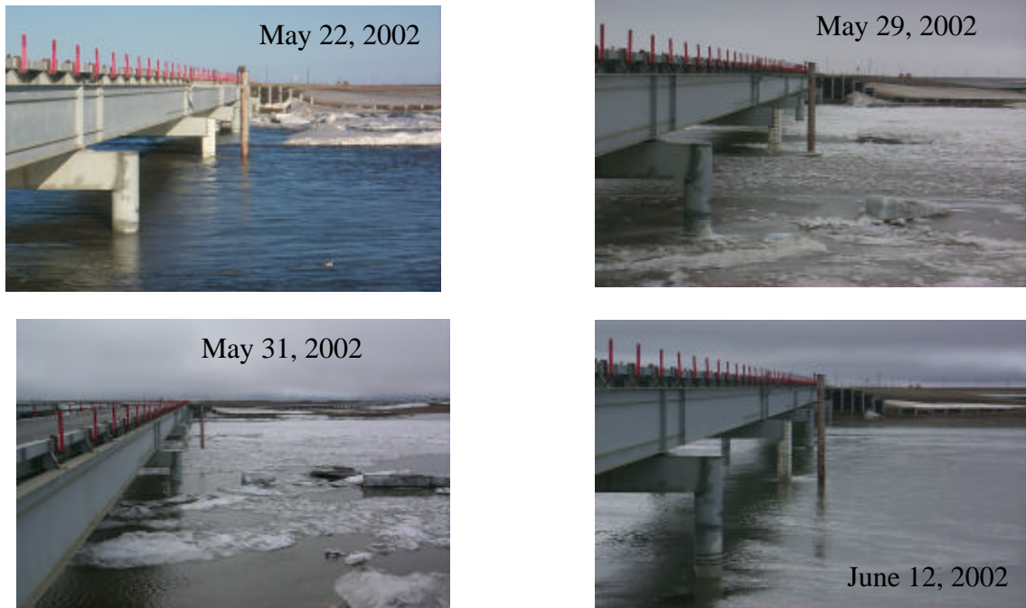
Figure 3-11. Sagavanirktok River flowing on May 22, frozen on May 29, and flowing again on May 31 and June 12, 2002 at bridge near Prudhoe Bay Operations Center.
