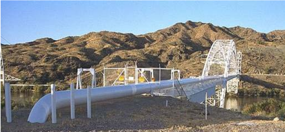
Pipelines like this above ground segment will benefit from the OPS-funded pipeline R&D projects.
