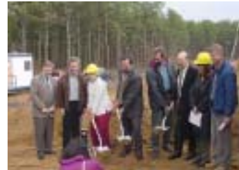
Construction begins on a new 12-unit affordable rental housing development in Wellfleet, MA.
