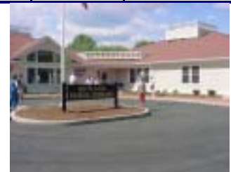
The Rutland Public Library was funded with a $2.9 million low interest loan from Rural Development.
