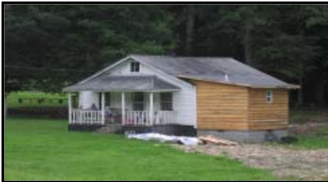
504 Repair Grant Butler, TN - Carter County
