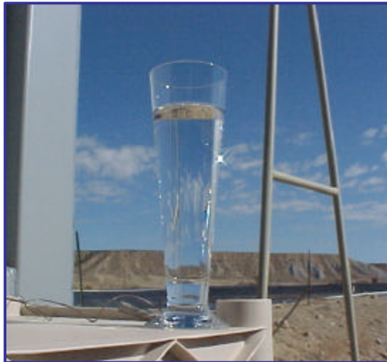
Crystal clear water -- The end product after reverse osmosis treatment.
