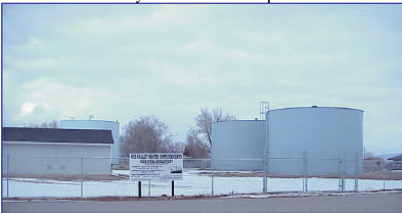
Midvalley Estates, Inc. Water Improvement Project for new well, tank and transmission lines. RUS Loan and Grant.
