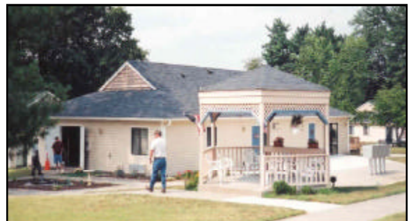
Above: Workers complete renovations to the office at Magnolia Place.
