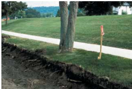
Figure 3.7. When the roots, stem, or branches are defective, a tree can become hazardous.
