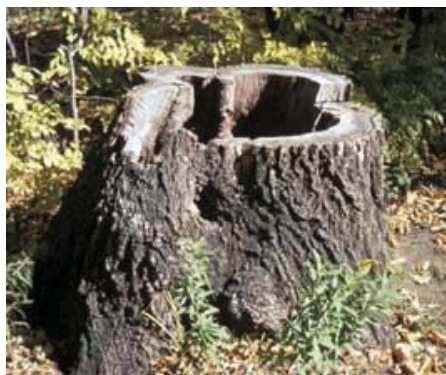
Figure 3.25. The outermost layer of undecayed wood is called the “shell.”
