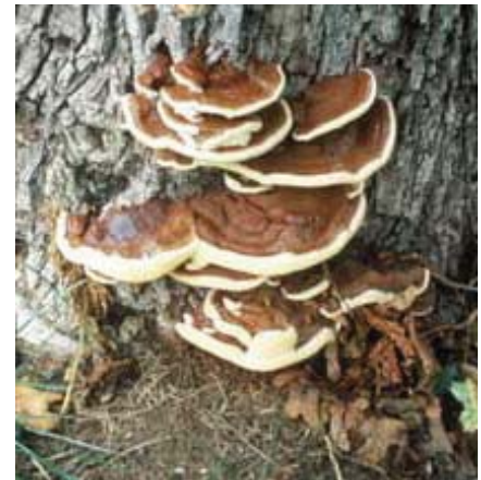
Figure 3.9. Fungal fruiting bodies indicate advanced decay.
