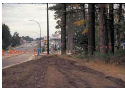
Figures 3.83-3.84. To estimate how much root damage was sustained, determine how much of the Critical Root Radius was disturbed.
