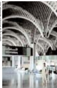
Reconstructed terminal at Baghdad International Airport
