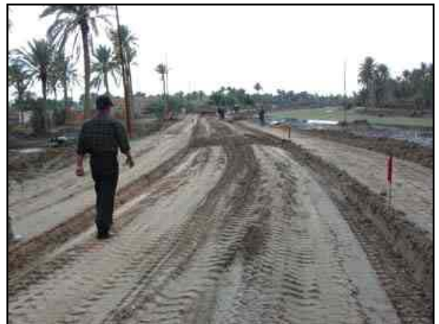
Repaving the main artery through Al Dibyanayah. Photo: USAID
