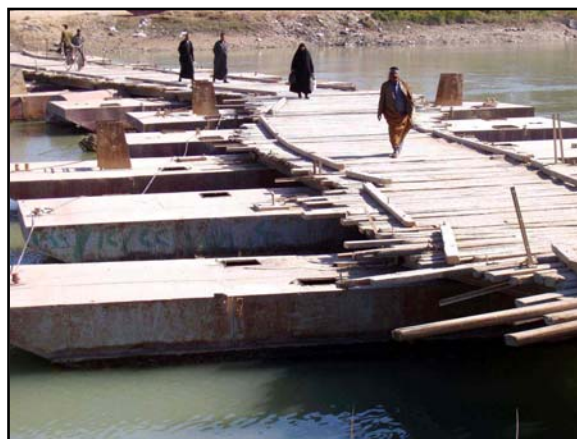
Al Abbasia Bridge in North Central Iraq connects 100,000 farm families to a market across the Euphrates River. Photo: USAID
