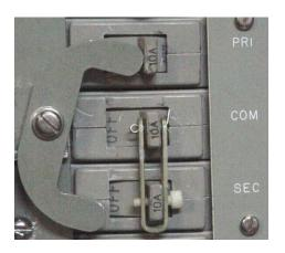
The alteration documents contain the procedure used to verify non-conducting bushings (NSN 9G-5970-01-094-1582) and screws (NSN 9G-5970-01-094-3317) installed. In addition, they outline the specifications for the warning sign required on the panel cautioning that removal of the non-conducting bushings and screws creates a potential shock hazard.
