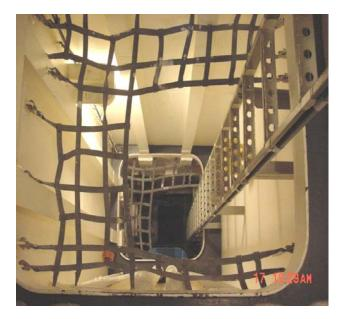
Most nets originally are manufactured and installed in accordance with specifications. However, problems arise when new nets are fabricated using the old nets as a pattern. The webbing stretches over time, and this causes each successive set of nets to become larger. Additionally, most nets are custom made for their intended location; putting them in another spot causes them to fit incorrectly.
