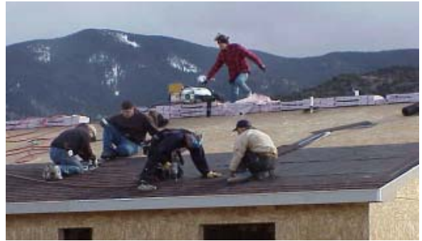
Families building a Mutual Self Help in Poncha Springs.
