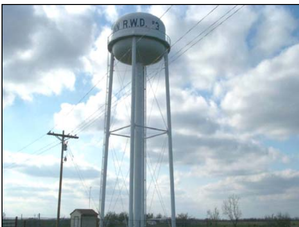
100,000 gallon tank for rural water district distribution system in eastern Kansas. This local rural water district serves over 300 Kansans
