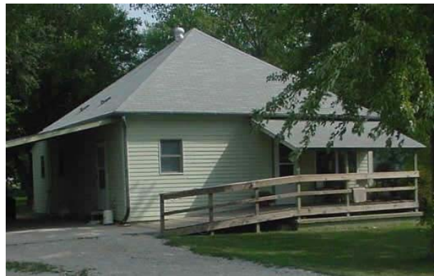
504 Repair loan in mid-central Kansas. Funds were used for new roof, new guttering, electrical repair and drywall
