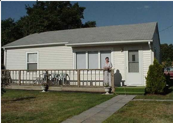
Funds were used for new siding, guttering, new windows, carpeting and vinyl throughout the home, new heating and air conditioning, and new roof for this home in central Kansas
