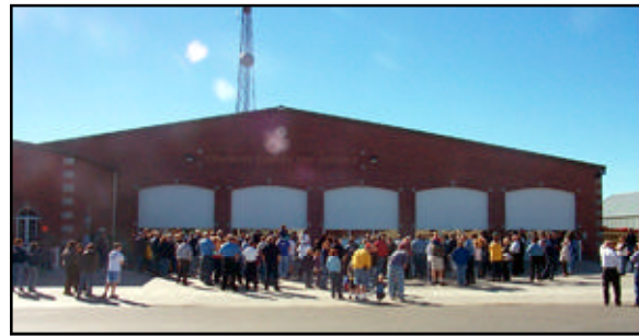
More than 150 people attended the open house of the new Franklin County, Idaho Fire District station. The new facility will also provide support for wildland fire operations within the county limits.
