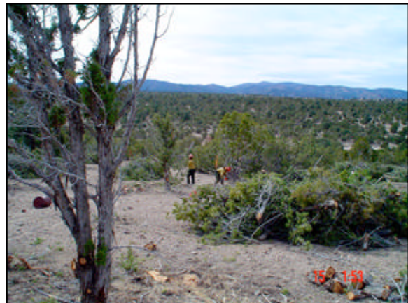
Crews in the Eureka area doing work on the project.
